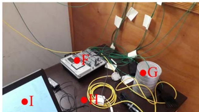
Fig. 5 Photograph of the experimental device in Haiti for roof measurements: F: Central measuring station (CR5000) where all sensors are connected; the green cables are thermocouples of type K allowing to measure the temperature. H: sensor to measure the sunshine (yellow cable). G: Cylinder in which a thermocouple is integrated to measure the dry air temperature. I: Computer connected to the central measuring station to record the data
