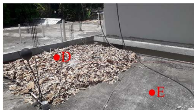
Fig. 4 Photograph of the roof in Haiti where the experiment was carried out, one part covered (D) with banana leaves and the other part not covered (E). The roof was subjected to the influence of solar radiation in order to test the thermal performance of banana leaves. In fact, the temperature of the bare concrete and that of the covered concrete has been measured. T sec : outside surface temperature of bare concrete (E), i.e., not covered with banana leaves. T sc : outside surface temperature of the concrete covered (D) with banana leaves, i.e., under the banana leaves
