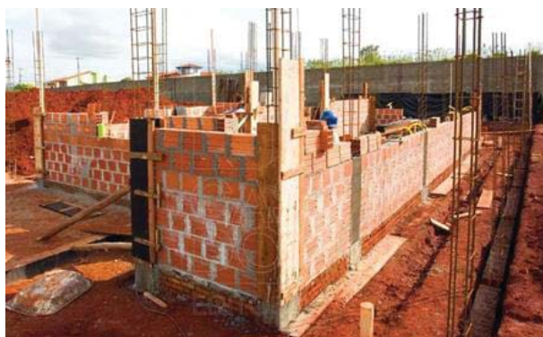
Fig. 2 Residential house made with reinforcement concrete and brick masonry
