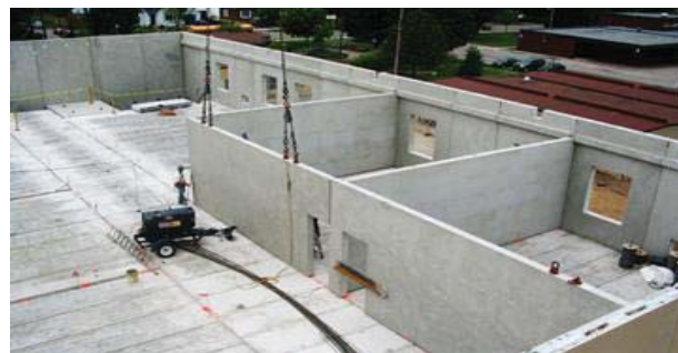
Fig. 3 Example of a building made with industrialized construction method in Colorado, USA
