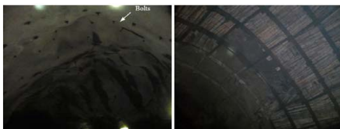
Fig. 2 Places with reinforced support in the ramp
