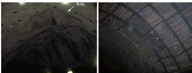
Fig. 2 Places with reinforced support in the ramp
