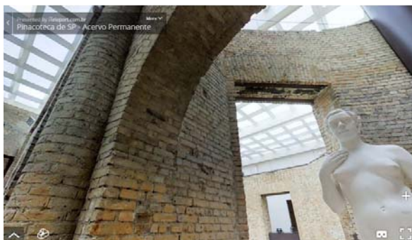
Fig. 11 Skylight in the central area in Pinacoteca of São Paulo [17]
