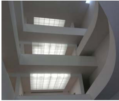
Fig. 5 Skylight on the last floor and artificial light systems on other floors; view from the atrium of the Iberê Camargo Foundation [13]
