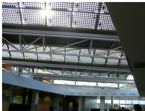
Fig. 1 Semi-transparent photovoltaic system of the Isofóton factory, Spain [4]
