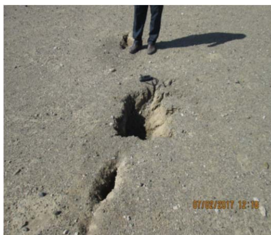
Fig. 5 Number of gaps and damage caused by it during a field survey
