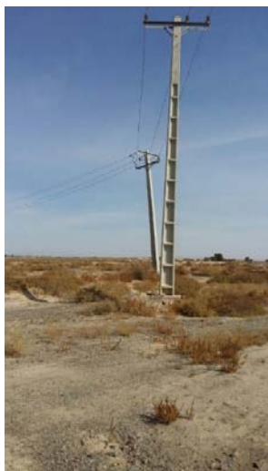
Fig. 3 Displacement of utility poles from vertical form to inclined form as a result of creep phenomena in the study area
