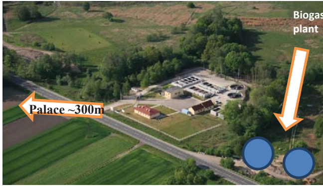
Fig. 7 Wastewater treatment plant with a biogas plant
