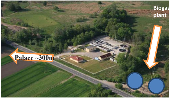
Fig. 7 Wastewater treatment plant with a biogas plant
