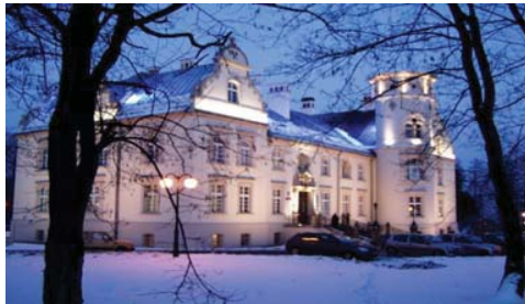
Fig. 8 Przyszwice palace complex with the health center, the Office of Civil Status and a kindergarten
