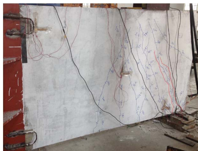
(b) Typical shear crack patterns for panel GS1 along the height of the concrete wythe
