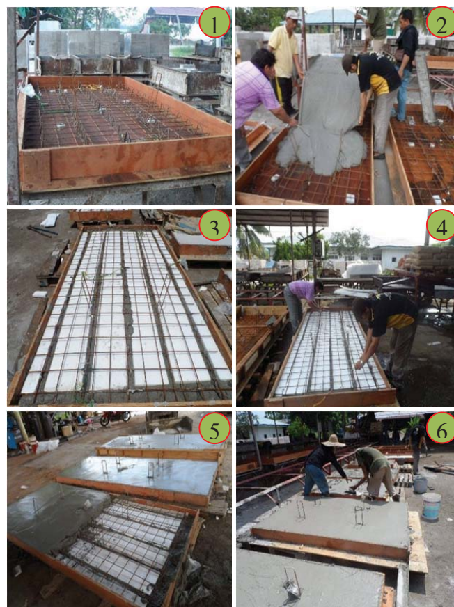
Fig. 3 Preparation, fabrication, and casting of PFCSP specimens
