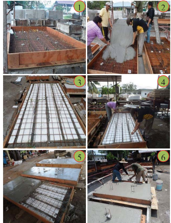
Fig. 3 Preparation, fabrication, and casting of PFCSP specimens
