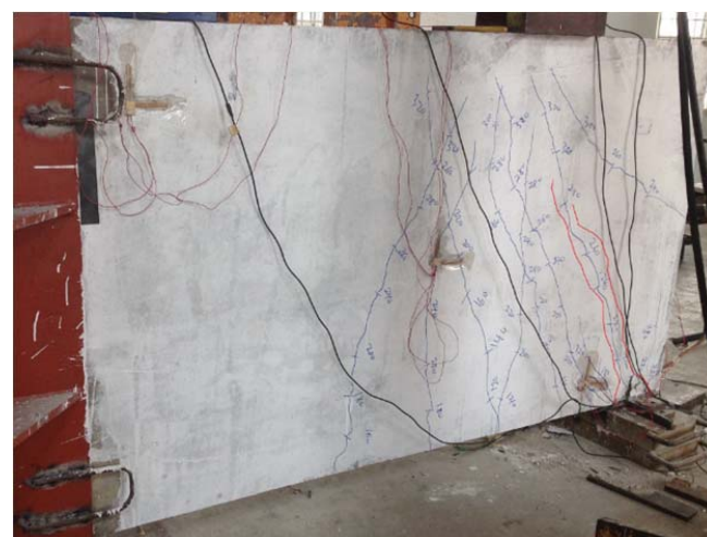
(b) Typical shear crack patterns for panel GS1 along the height of the concrete wythe
