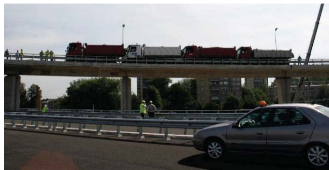
Fig. 4 South bridge overpass 5-2
