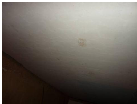
Fig. 2 Test slab after the 186 min of fire resistance testing – surface loaded by the high temperature
