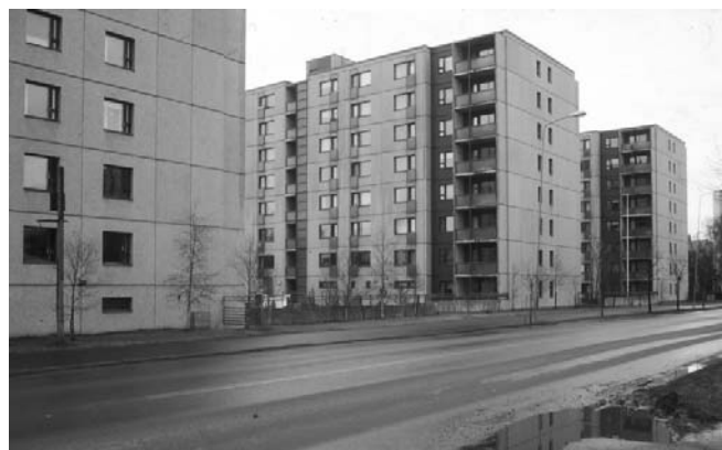
Fig. 1 Typical Finnish concrete apartment buildings from the early 1970's. The buildings have a load bearing bookshelf frame, non-load bearing facades of concrete sandwich elements and self-load bearing balconies
