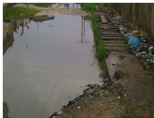
Fig. 1 Abrupt truncation of drainage, that resulted in flooding
