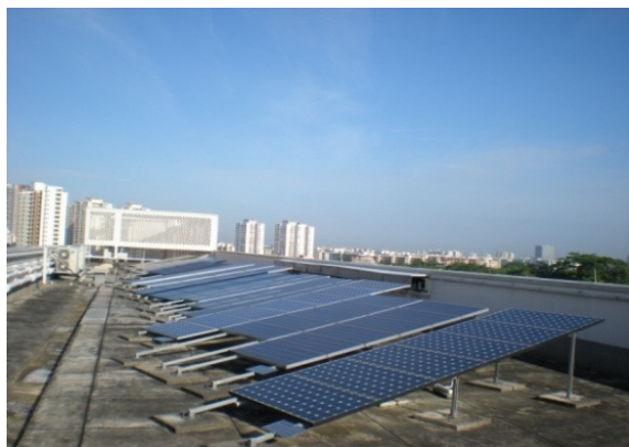
(b) After installation of PV systems
