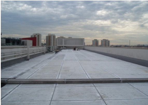
(a) Before installation of PV systems
