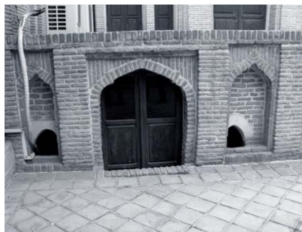
Fig. 5 Entry of Shavadan from the Yard
