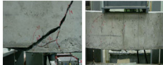
Fig. 14 Anchored aluminum strengthened RC structure failure mode
