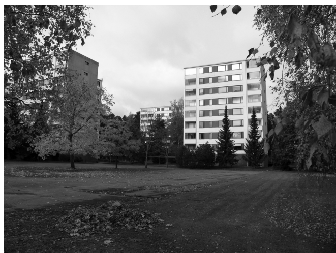
Fig. 1 A significant number of suburbs were constructed in Finland in the 1960's and 1970's
