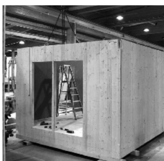
Fig. 6 Fabrication of CLT module elements
