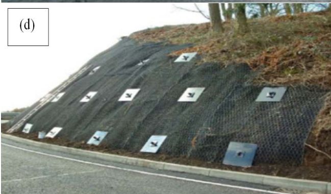
Fig. 5 Soil Nailing Method
