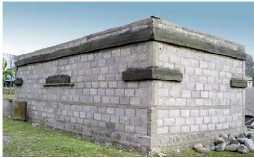
Fig. 7 (a) Roof band beam and wall L-stitches
