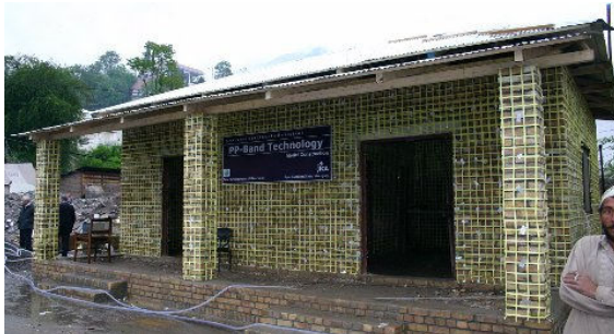
Fig. 7 (b) Polypropylene band reinforcing
