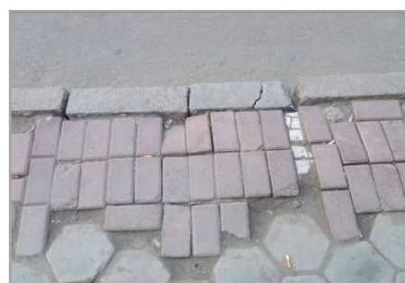
Fig. 16 (a) Damaged pavement on the Ceramic Street logos on the Ladies' Street
