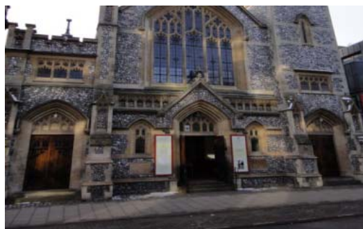
Fig. 2 (a) Landscape elements—roadside buildings
