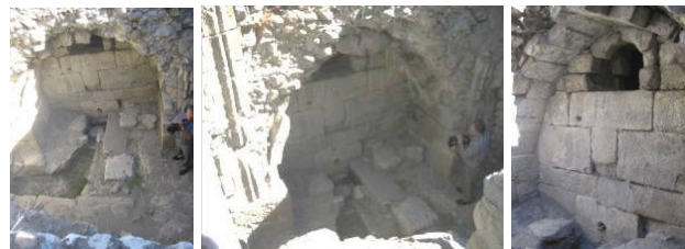
Fig. 7 Fountain's north façade
