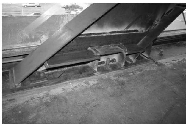
Fig. 13 Photo of constructed shearlink
