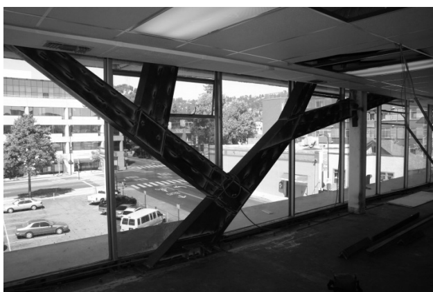
Fig. 14 Photo of frame under construction
