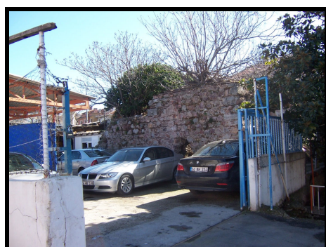
Fig. 9 Bath's south facade - 2014
