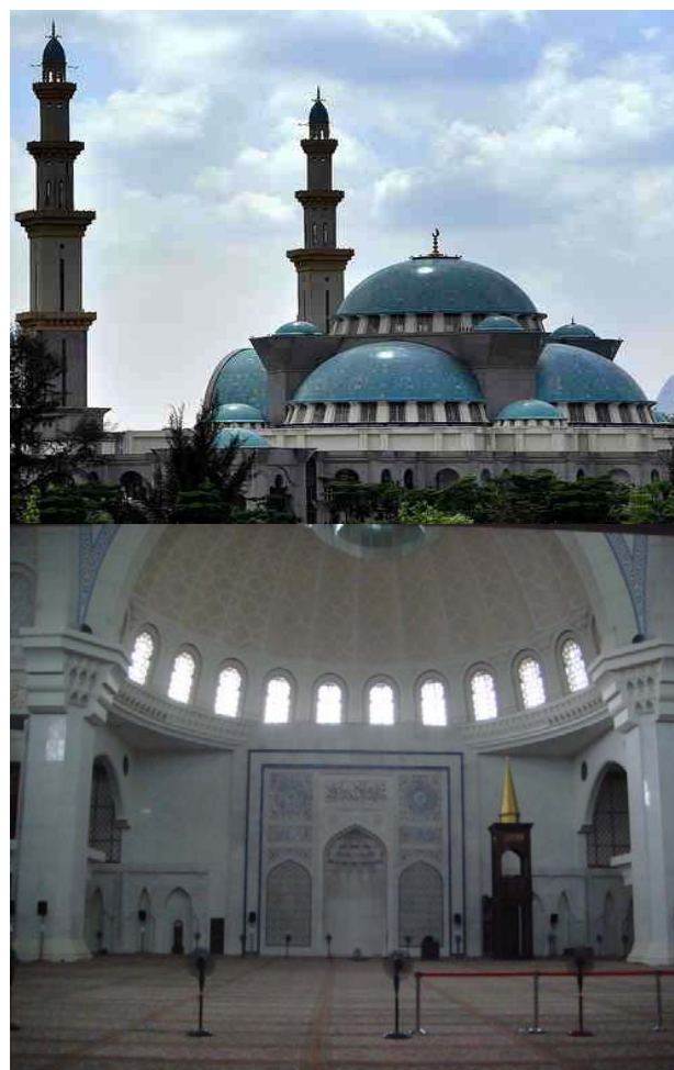
Fig. 4 Exterior (Top) and Interior (Bottom) of Masjid Wilayah
