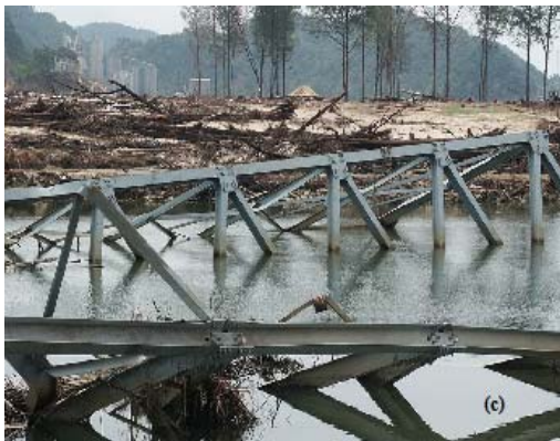
Fig. 2 Bridge damage due to tsunami attack in Banda Aceh (a) Total Wash-Away of Deck [7] (b) Excessive Deck Displacement [12] (c) Damaged steel truss bridge with damaged cement plant in the background in Lhok Nga, Banda Aceh
