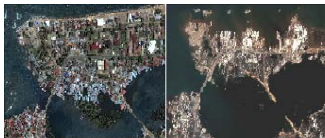
Fig. 1 Effects of tsunami 2004, along coastal line and bridge structures in Banda Aceh, Indonesia
