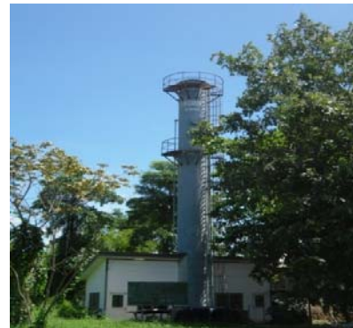
Fig. 5 The design of the Department of Local Administration cooperated with the Metropolitan Waterworks Authority
