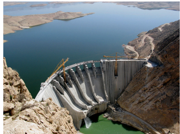
Fig. 3 Salman Farsi (Ghir) dam is a 125 m high concrete gravity arch dam within the Ghareh Aghaj River (northeast view)
