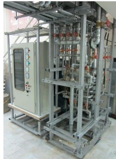
Fig. 6 Picture of inverter box with some air cooling lines (MFL-TMU)
