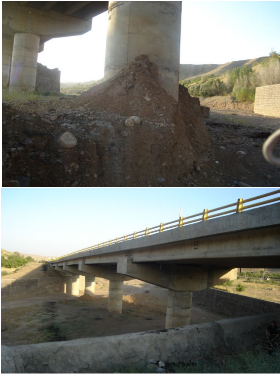
Fig. 1 Span bridge situated in 11+406km of the Marand-Soufian route
