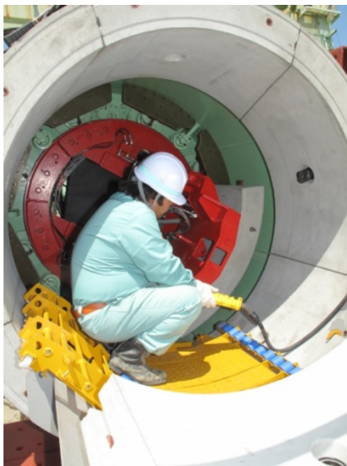
Fig. 6 Secondary lining applied RC segment – assembly
