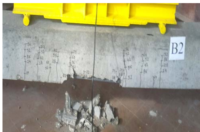
Fig. 5 Typical splitting failure for beam specimens without confining transverse reinforcement
