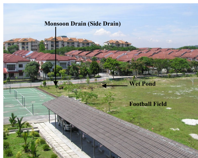
Fig. 2 Catchments of the constructed mini wet pond
