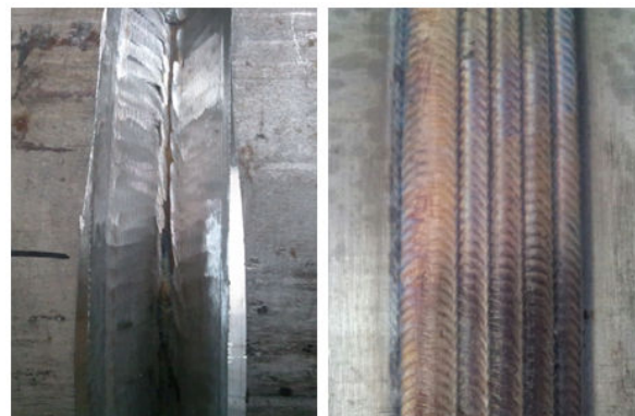
Fig. 9 Before and after welding quality of Duplex steel
