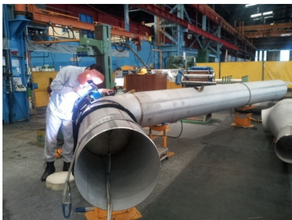
Fig. 8 Stainless steel pipe welding in DSME shipyard
