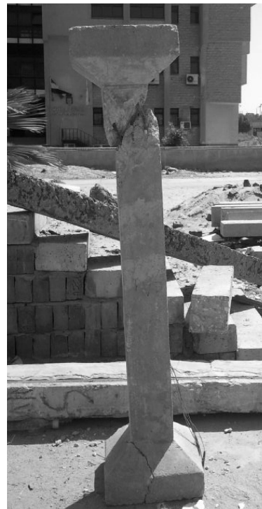
Fig. 18 Failure mode of axially loaded column
