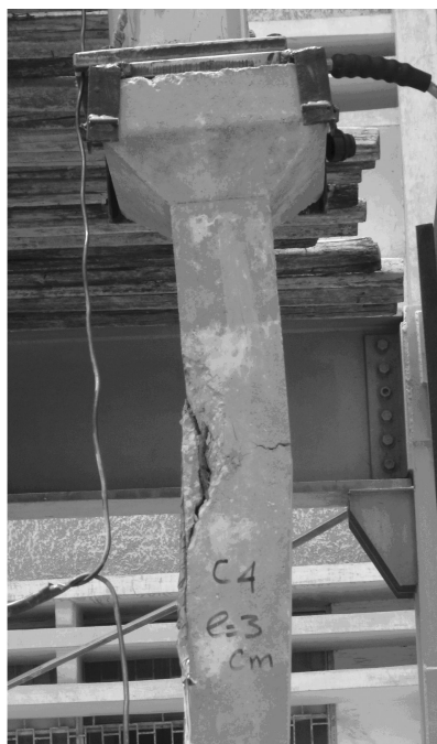
Fig. 19 Failure mode of eccentrically loaded column
