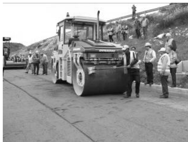
Fig. 3 Roller compacting SFR-RCC layer during demonstration day.
