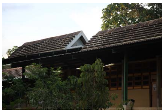
Fig 9. Campus UFAM, Manaus. Concrete roofing, with openings to allow air flow and improved thermal pefromance, while protecting from intense solar radiation and rains.
