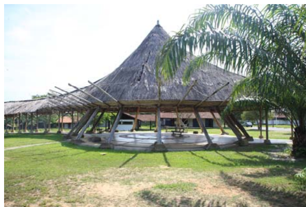
Fig. 10. Aldeia SOS, Manaus – Brazil. The use of 'piacava' another natural fibre commonly used by indigenous people in the Amazon region, and reincorporated by the architect Severiano Porto for this project in 1992.
