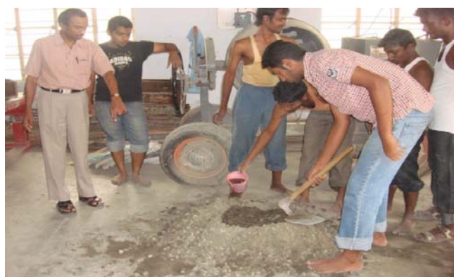
Fig. 1 Mixing of Concrete for Casting of Beam Specimens
