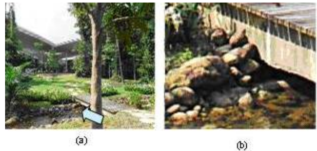
Fig. 2 (a) View from 10m from the pebbles (as shown by arrow) (b) view during a zoom to the pebbles
