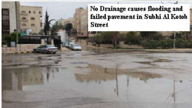
Fig. 3 (a) Example Problems of the roadway drainage systems in Site 1
