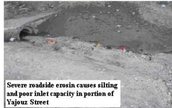
Fig. 5 Example Problems of the roadway drainage systems in Site 3
