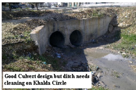
Fig. 4 Example Problems of the roadway drainage systems in Site 2
