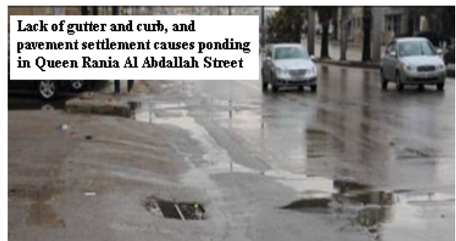
Fig. 3 (b) Example Problems of the roadway drainage systems in Site 1
