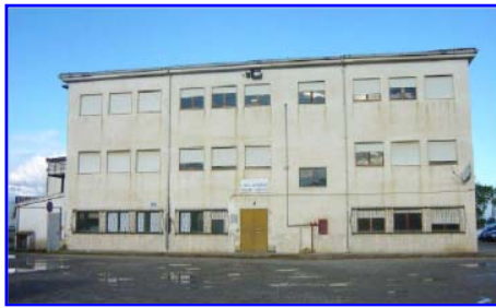
Fig. 1 View of the main façade of the building
