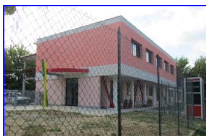
Fig. 20 View of the building after the completion of the retrofit and architectural renovation works
