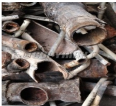
Fig. 16 Rusty broken pipes
