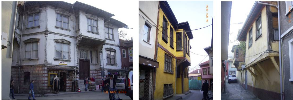
Fig. 11-13. The use of buttresses at the houses Photos: Özlem Köprülü Bağbancı, 2006
