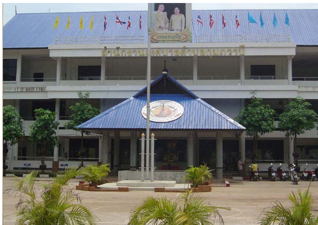
Fig. 2 The Municipal Office of sub-district Kumphawapi
