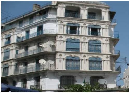
Fig. 2 Stone masonry building in Algiers with irregular structural layout
