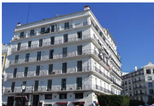
Fig. 1 Stone masonry building in Algiers (multi-family residential buildings containing a commercial ground floor and five stories)
