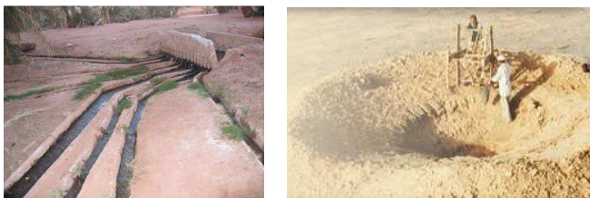
Fig. 3 Appearance (left) and Excavation (right) of Qanat
